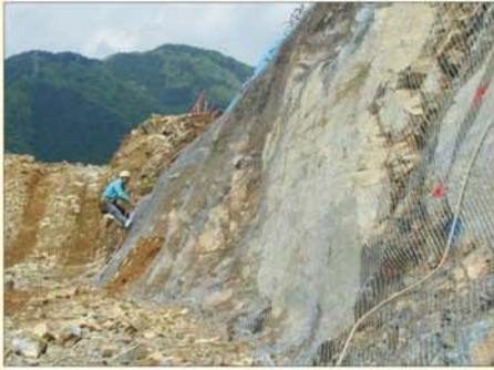
1. Laying Wire Mesh
