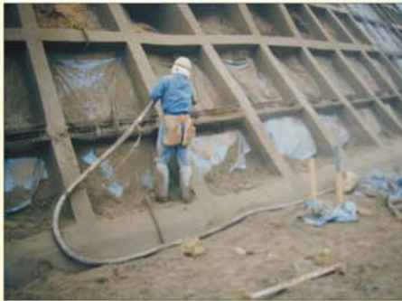
4. Wet Spraying Cement/Sand Mortar
