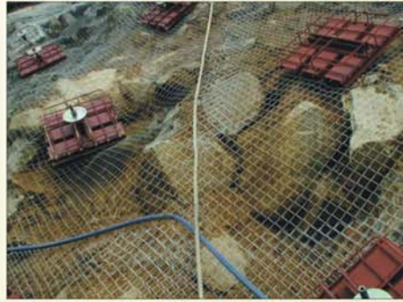
2. Installation Soil Nail Head
