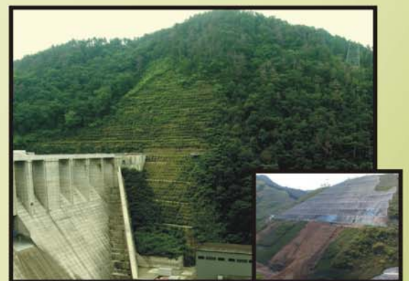
After and After the Works
