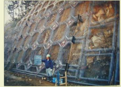
3. Installation of Reinforcement Bar
