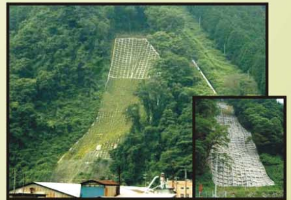
Hydromulching Cover and Shotcrete Cover
